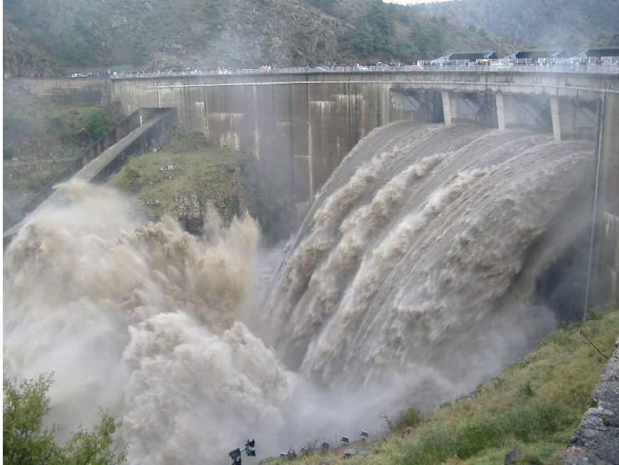
Loire at Grangent, november 2008.
