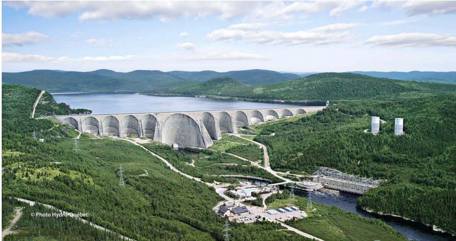
Daniel-Johnson Dam. Source: Hydro-Québec ( hydroquebec.com ) autorisation for non-commercial reuse
